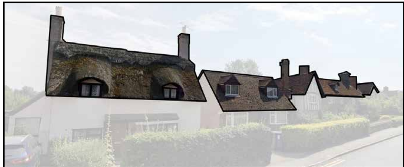
Arlesey Road. Images above show positive examples of roofscape articulations
