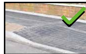
Uninterrupted footways over driveways
