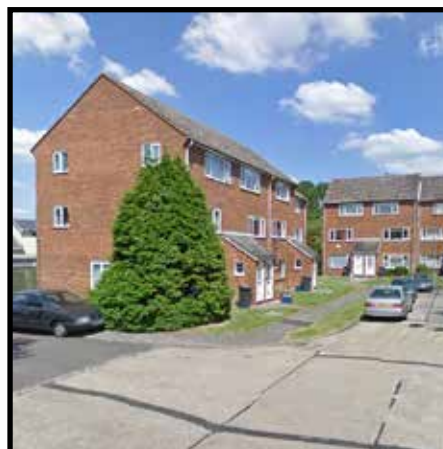
B Rarely, terraced houses that look like small flat buildings or flat buildings as part of retirement homes.
