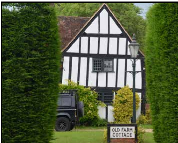
Exposed timber frame with painted brick infill and ceramic tile roofs
