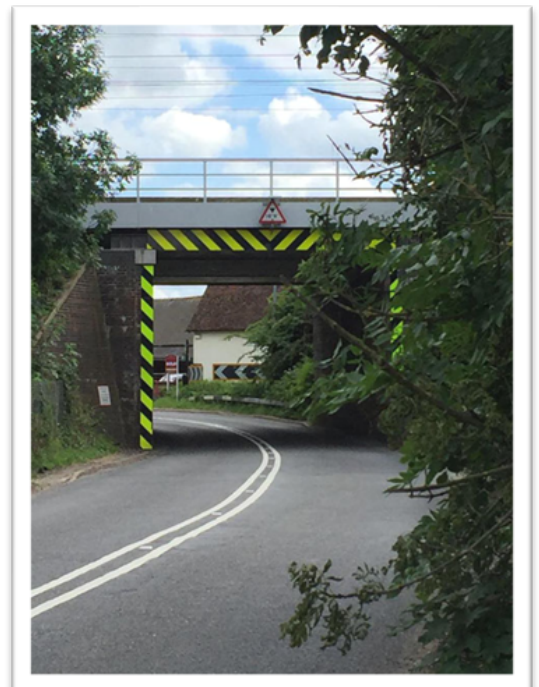
Cadwell Bridge - a major pedestrian safety issue
