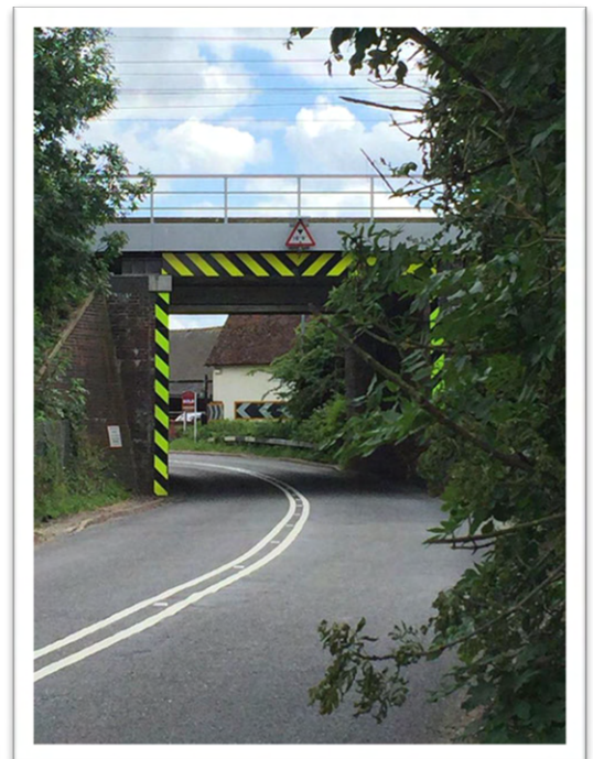
Cadwell Bridge - a major pedestrian safety issue
