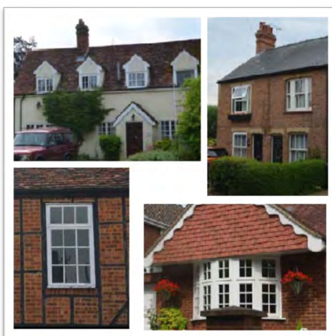
Typical construction features in the village, from years past.
