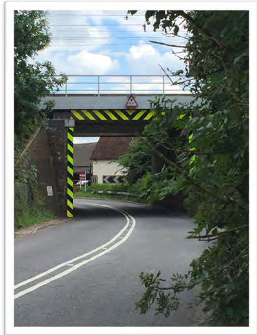
Cadwell Bridge - a major pedestrian safety issue
